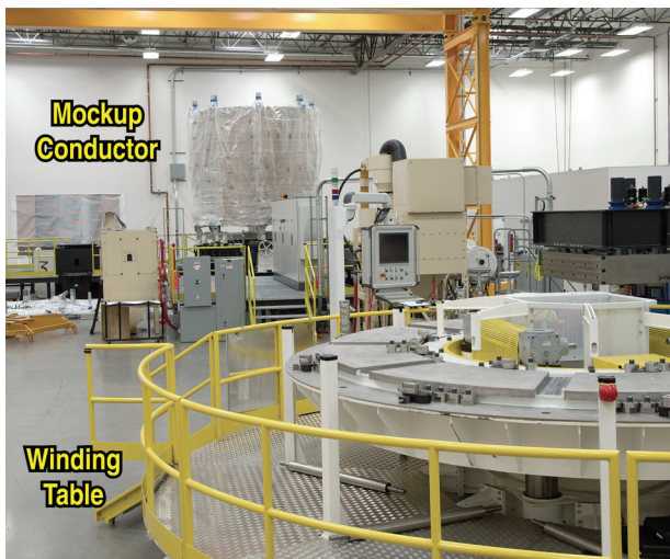
Fig. 1. Tauring's winding system installed with 900 m of mockup conductor loaded onto the de-spooler.
