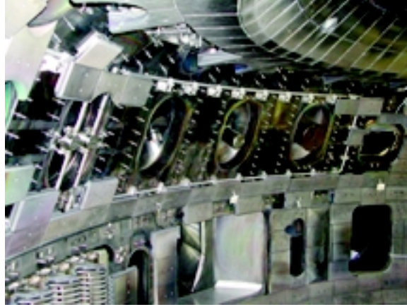
Fig. 2. Installation of two prototype I-coils in DIII-D, October 2001.
