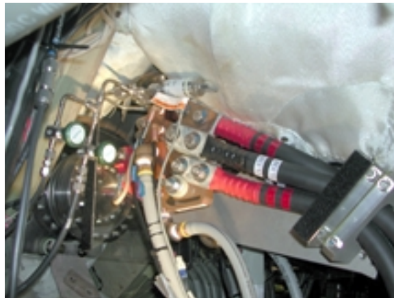
Fig. 7. Electrical power and fluid connections to a pair of lower I-coils. The transition between coaxial lead and quadrupoled power cable produces some uncancelled I \times B forces.
