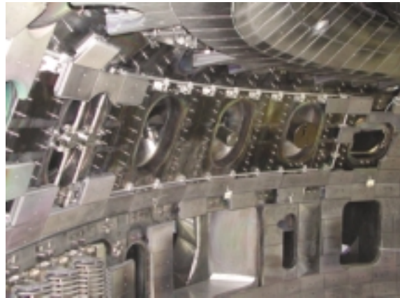
Fig. 1. Installation of 2 prototype 1 coils, October 2001.
