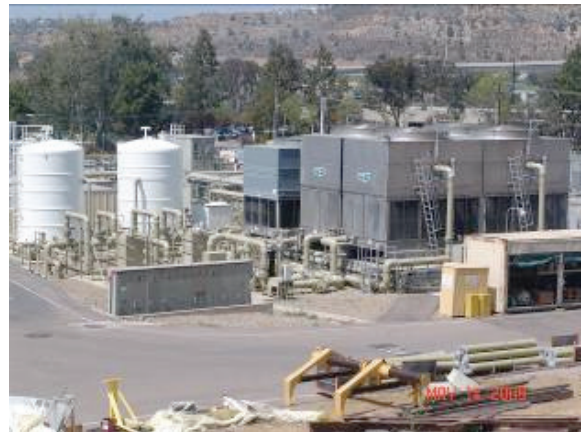
Figure 1. New stainless steel Evapco cooling towers with new PVC piping.
