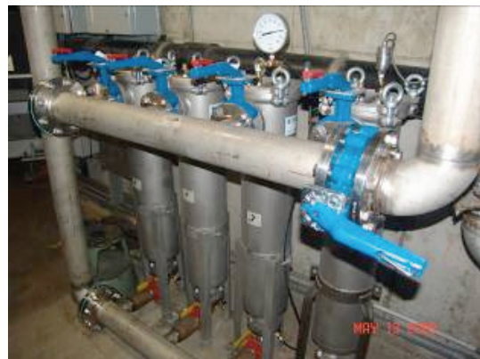
Figure 6. Eaton Flowline Multi-Housing Bag Filters.
