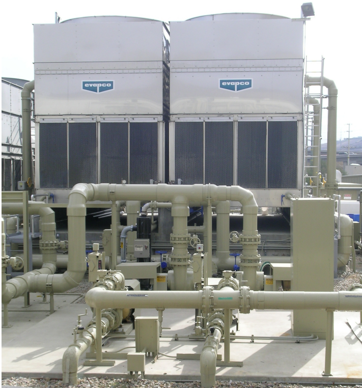
Cooling towers installed
