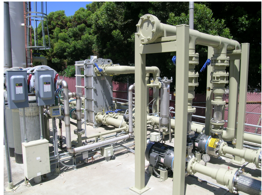
Upgraded ECH HX and Pumps
