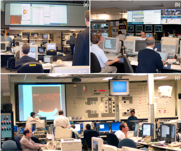
Figure 1. The control rooms of NSTX (a), DIII-D (b), and C-Mod (c) with shared display walls being used to enhance collocated collaboration. On the DIII-D display is also video from remote collaborators in Europe who were participating in that days experiments.
