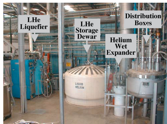
Figure 1. DIII-D cryo system’s liquefier, helium storage dewar, wet expander and distribution boxes.
