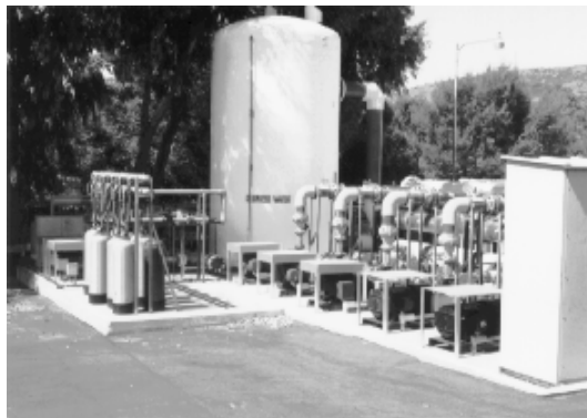
Fig. 3. Auxiliaries Low Pressure Cooling Water System.
