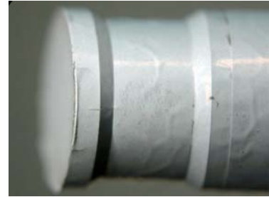
Fig. 3-46. A defective aluminum coating showing wrinkles and cracks.
