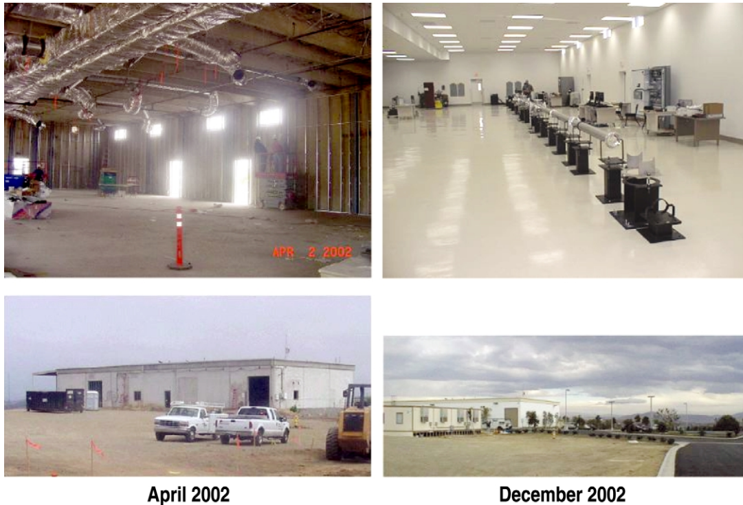
Fig. 3. The IFE target fabrication and injection facility before and after renovation.
