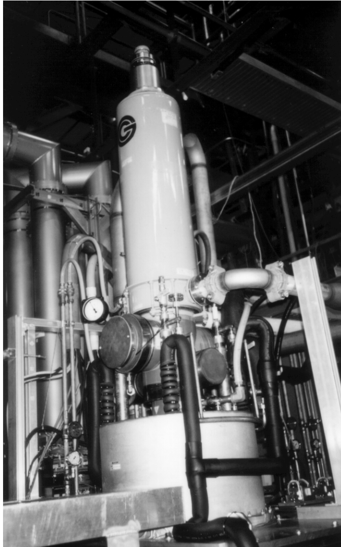
Fig. 6.1-1. 110 GHz GYCOM gyrotron installed in DIII-D ECH vault.
