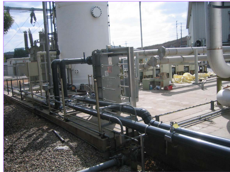
Installation of new ECH heat exchanger
