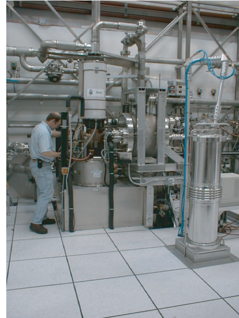
Gycom gyrotron Boris installed in the new ECH gyrotron vault
