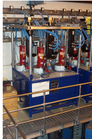
Klystron Assembly 8-16 @ 250 kW each
